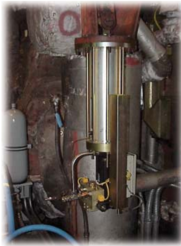
Reheat stop valve conversion
